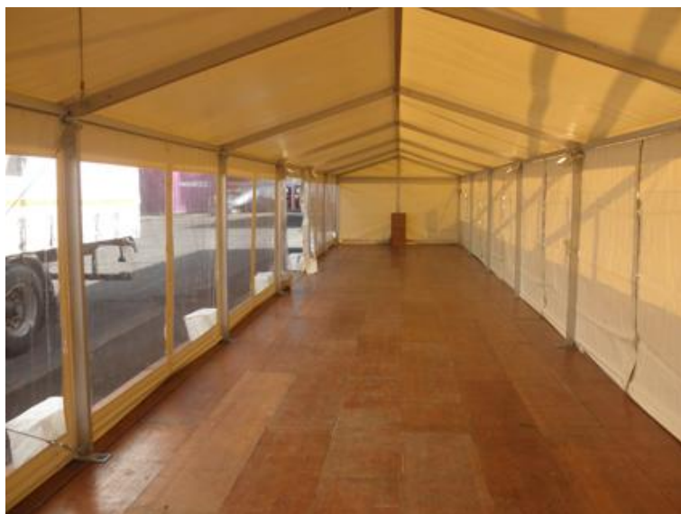
Structure 4m x 18m, surface 72m 2 , buvette manifestation
